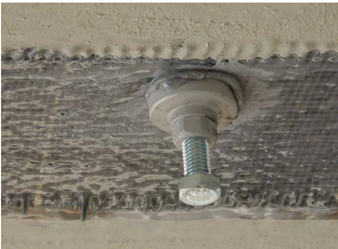
Figure 14: Pull-off plug installed on the bridge deck
