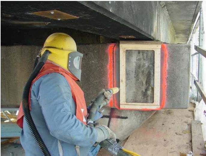
Figure 12: Surface preparation by sandblasting.
