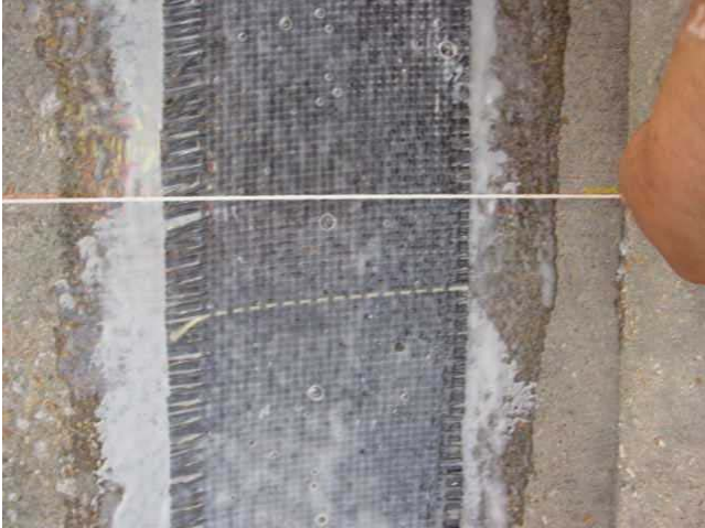
Figure 11: Alignment errors of 7.2 and 0.9°, respectively.
