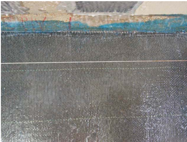
Figure 3: FRP sheets with yellow tracer and overlain by white chord.
