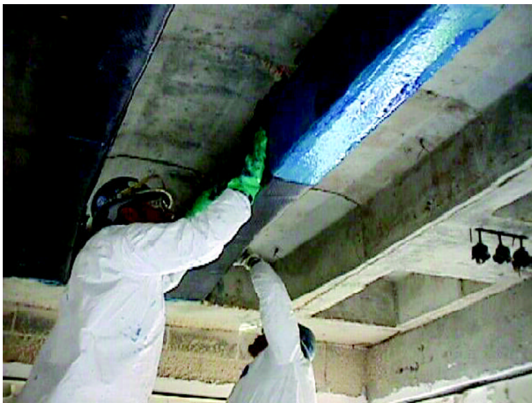
Fig. 1: Application of FRP sheet on one-way joist
