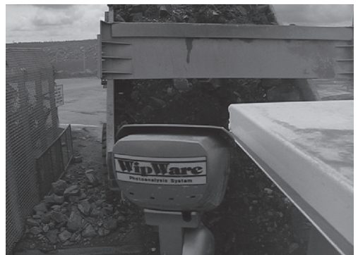
Figure 13. Imaging at a truck dumping station at Municipal Quarry in Bedford, Nova Scotia, Canada.
