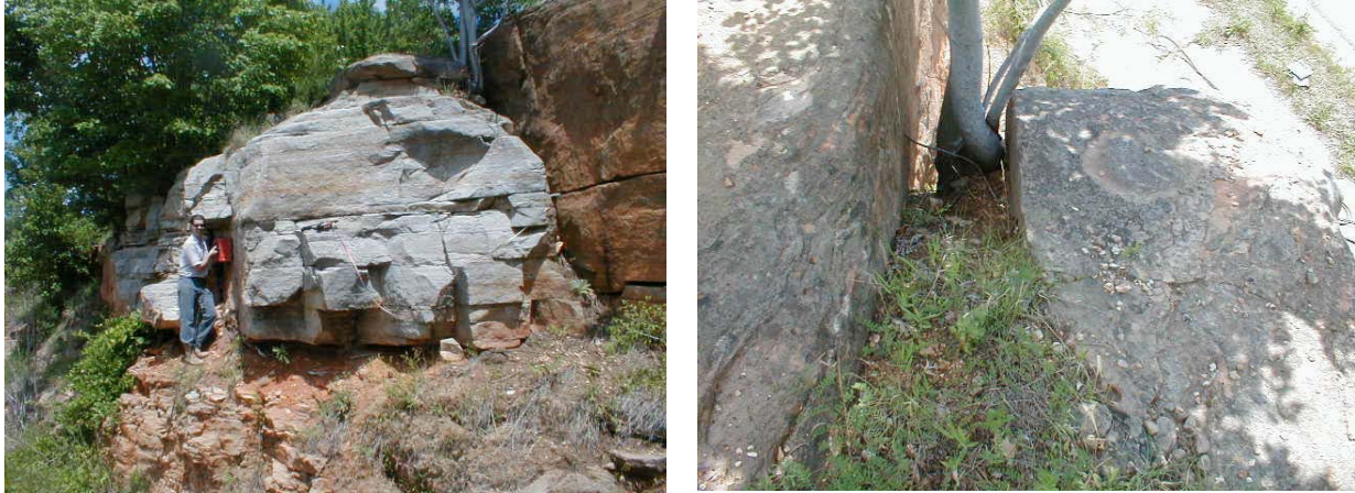
Figure 12. Site 4 with a 12" soil filled vertical joint, 10' deep into the rock'.
