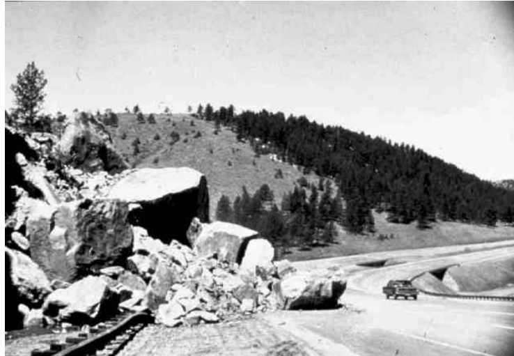
Figure 1. Example of a rock failures causing obstruction of a roadway.
