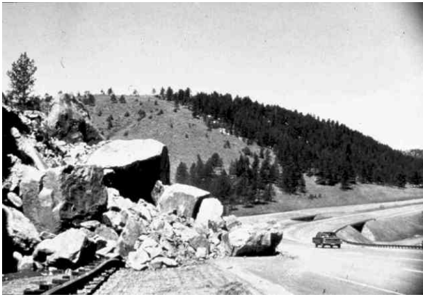
Figure 1. Example of rock failures causing obstructions in roadways
