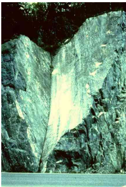
Figure 3. Example of wedge, planar, and toppling failures along road cuts.
