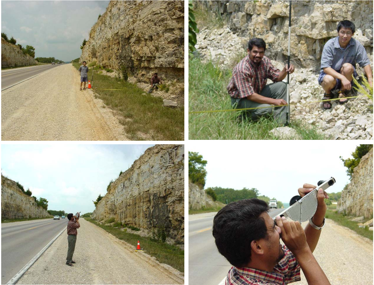
FIGURE 8 Manual measurements of road widths, ditch widths and depths, and slope heights and angles.
